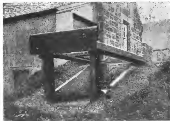
AN EASILY CONSTRUCTED AUTOMOBILE PIT.
